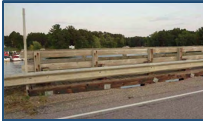
CTH Z Pedestrian Bridge
